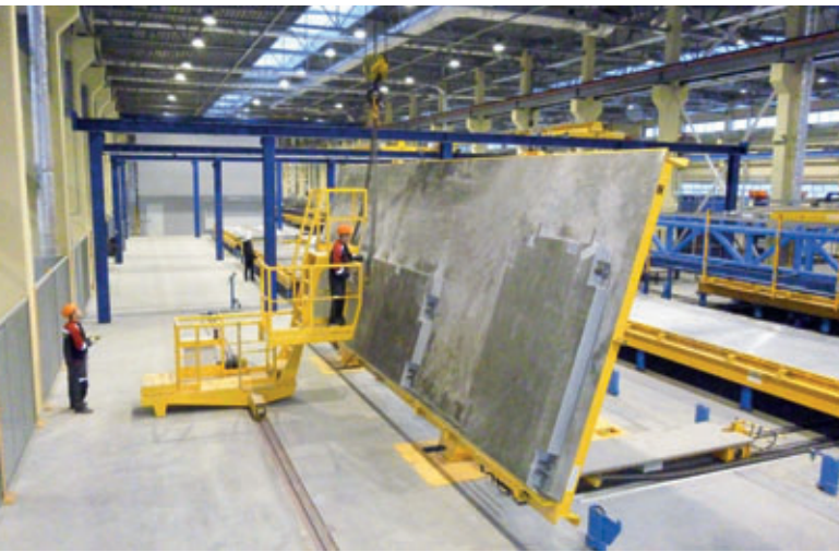
A tilting facility brings the pallets into an almost vertical position for the removal of the finished wall elements. Mobile steps facilitate the process for the operator.
