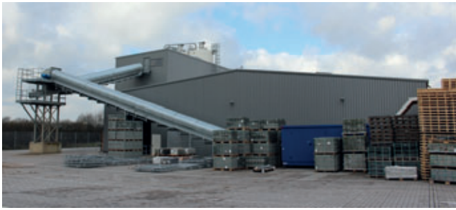
The aggregates are transported via two 800 mm wide conveyor belts (34 and 22 m long) to the highest level of the mixing tower, which is integrated in the hall.
