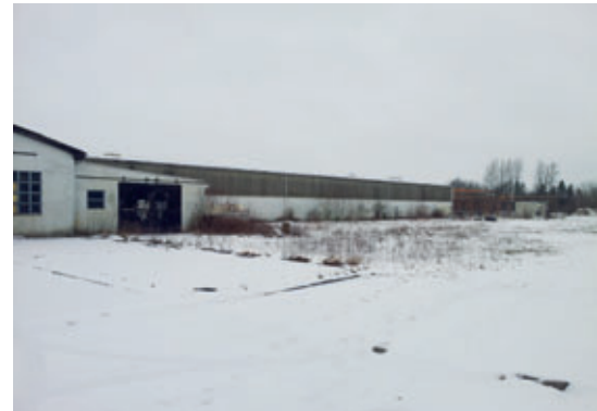
Lithonplus turned this old hall into a state-of-the-art production facility.
