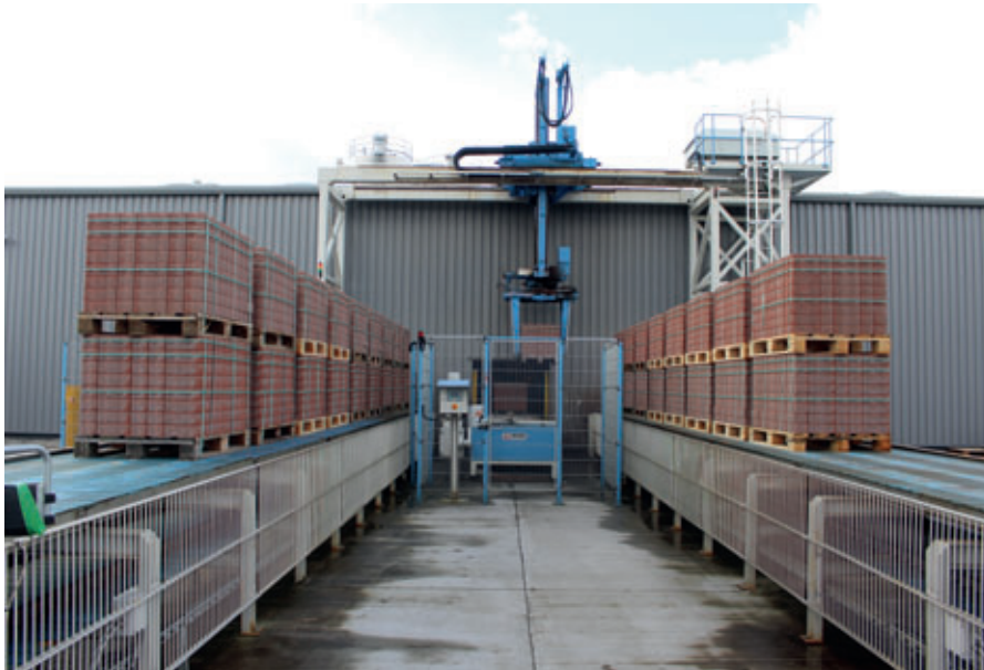
A robot crane takes up the stone packages together with the wooden pallet and sets them down alternatively on the buffer conveyors arranged symmetrically on the left and right. In the process the stone packages are doubled, which means that two complete stone packages are always placed one on top of the other.
