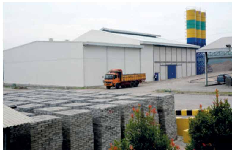
The new plant is located about 100 kilometers SE of Jakarta
