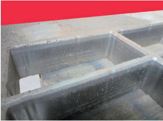
Wear in the compaction area
