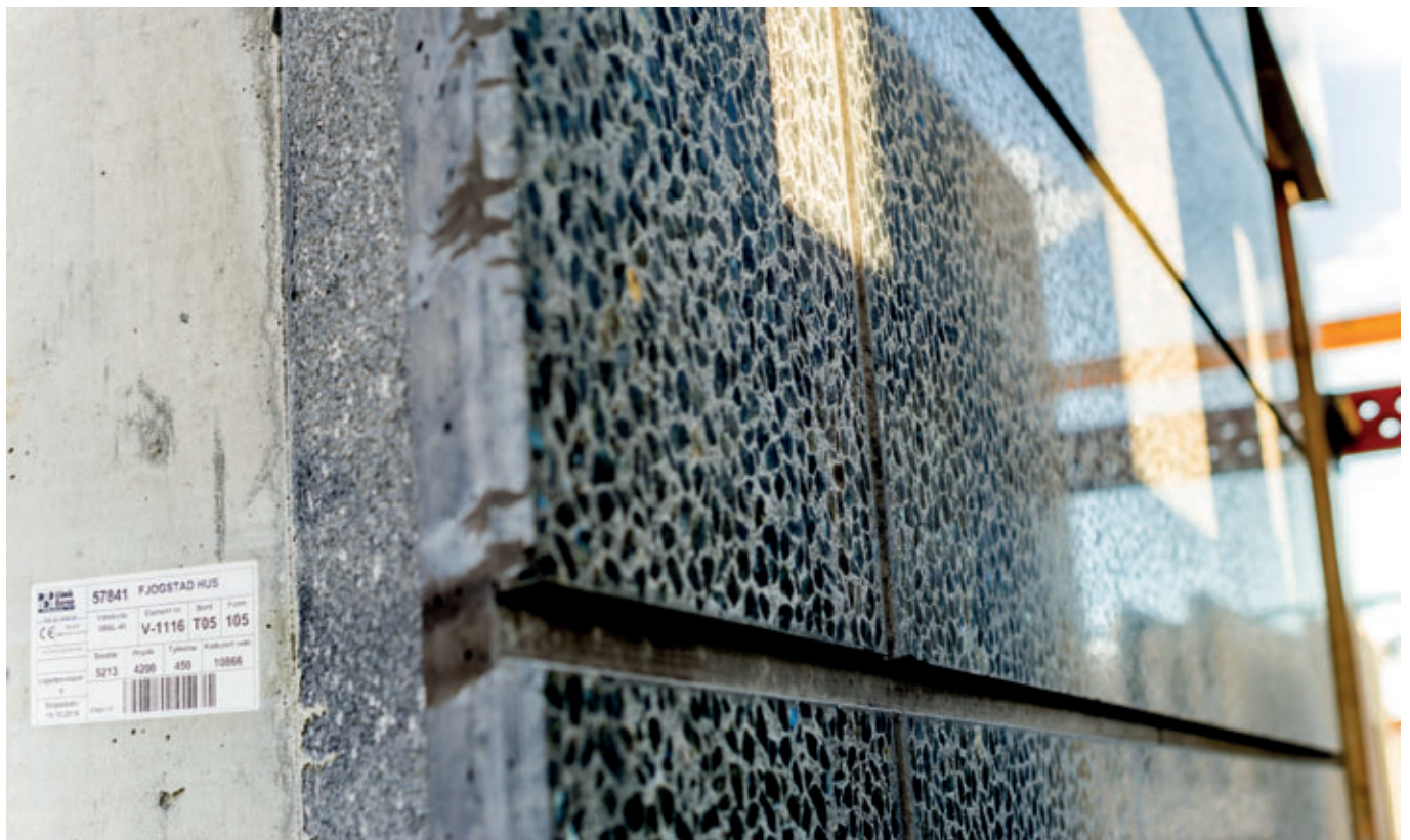
Detailed view on a surface treated precast concrete element
