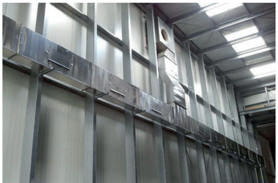
Picture of transfer car area taken with chamber temperature of 35°C (100°F) and relative humidity of 90%. The floor and walls are very dry and there is not any fog or haze which is important for the operation of transfer cars using laser positioning.
