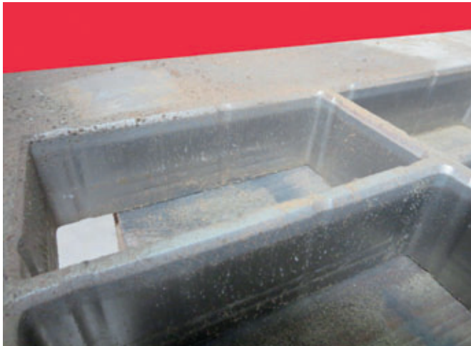
Wear in the compaction area
