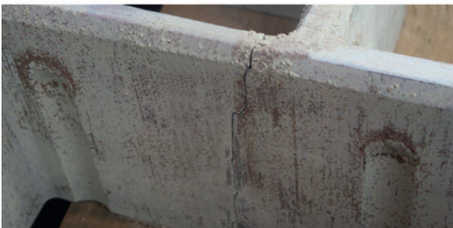
Overstressing/cracks
