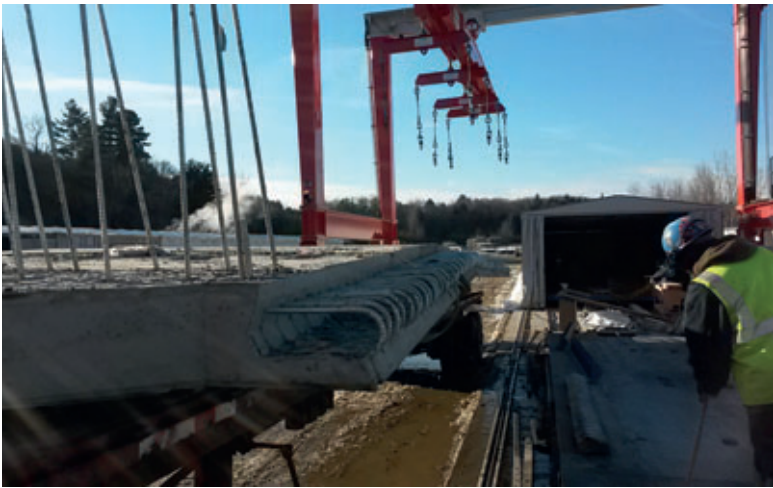
Precast concrete deck panel for the new bridge.
