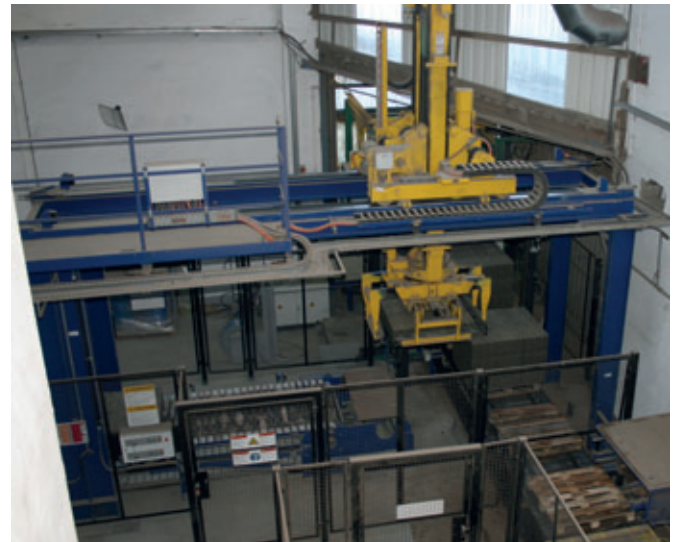
Packaging the pumice concrete blocks on wooden pallets
