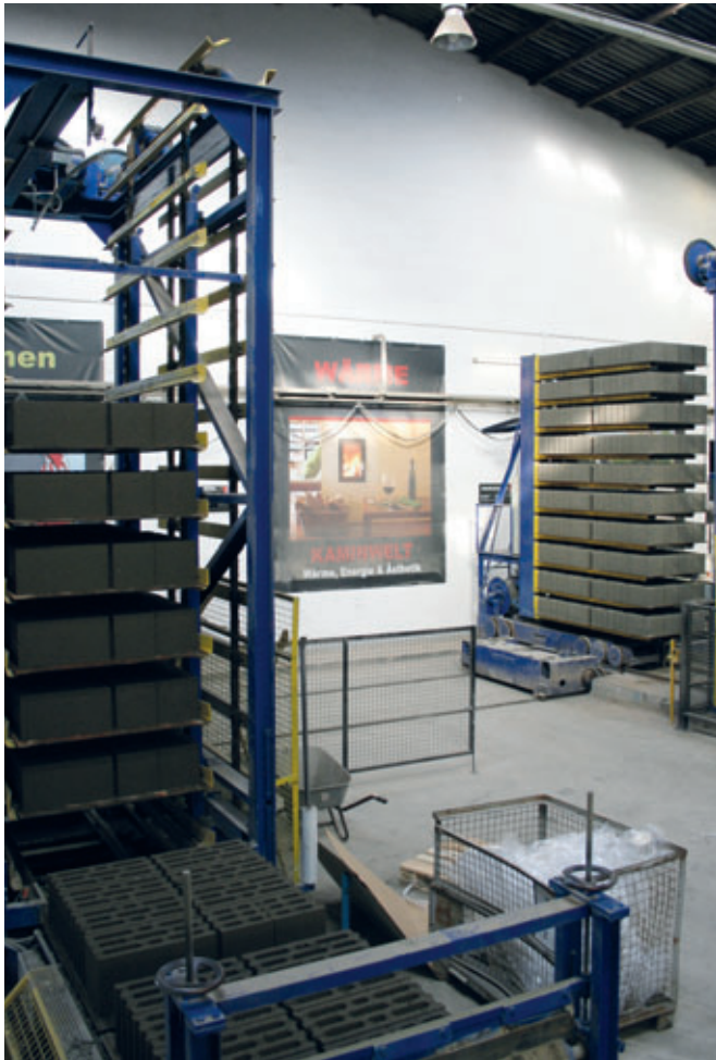
Both the elevator and lowerator as well as the finger car were modernised.
