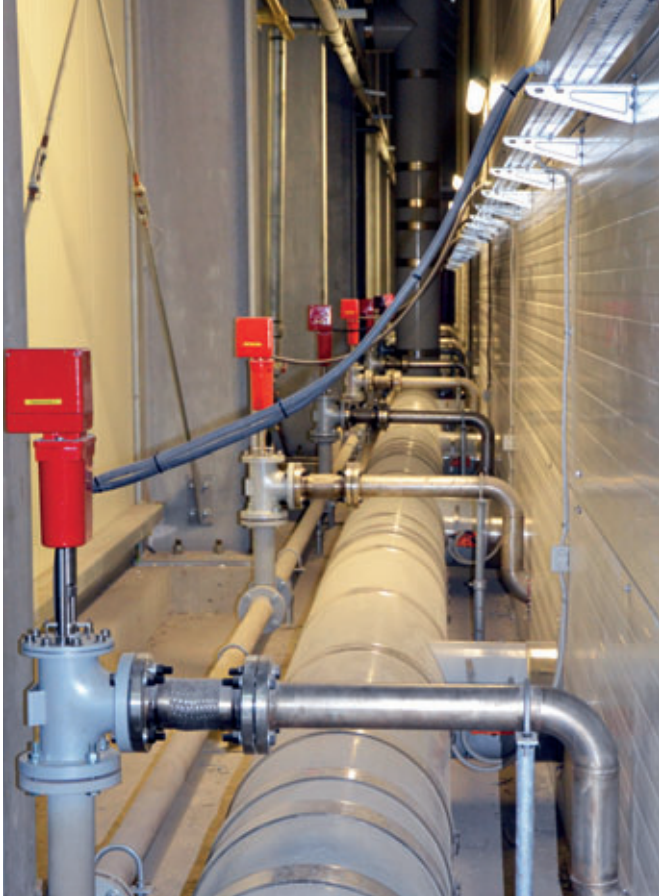
Piping gangway on the rear side of the slab rack with vapour pipe, a valve for each curing chamber and the air distribution pipe.
