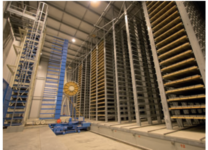
Drying chamber with racks from Rotho in the new Vibor-S plant in Russia: total capacity 8000 boards
