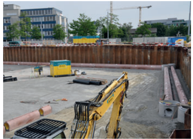
The progress of construction work – laying, filling, compacting – was significantly increased through the use of Perfect Pipe with connector in this major construction site in Zurich as described
