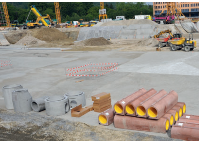
In addition to the concrete-plastic composite pipes, Beton Müller also supplied customised Perfect manhole bases to Zurich
