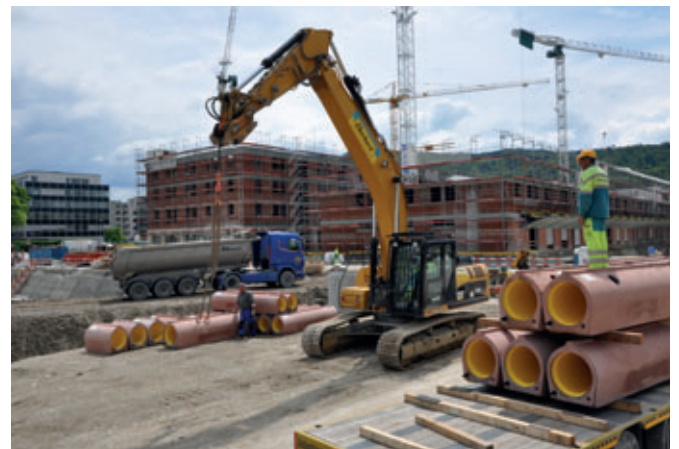
The anchors cast firmly in concrete ensure safe handling of the robust concrete pipes, with or without liner
