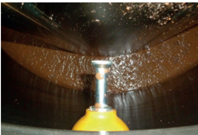
By filling the moulds with fluid concrete, built-in components such as transport anchors are completely encased in concrete
