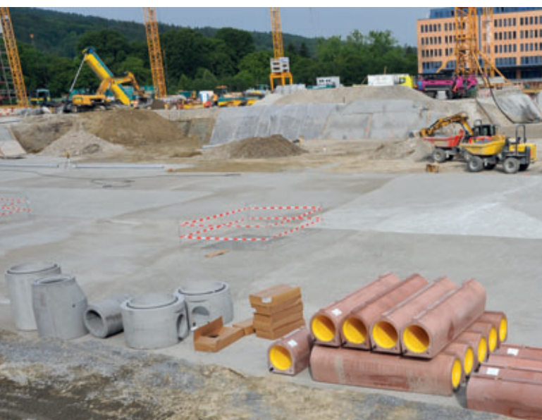
In addition to the concrete-plastic composite pipes, Beton Müller also supplied customised Perfect manhole bases to Zurich
