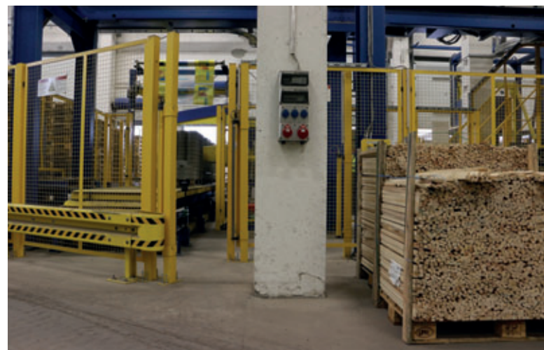
Safe working without loss of time – thanks to the light barriers the strips can be positioned reliably without disturbing the overall plant sequence
