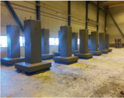
Foundation blocks with foot
