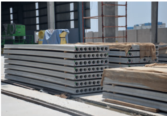
Hollow-core slabs and precast walls in stockyard
