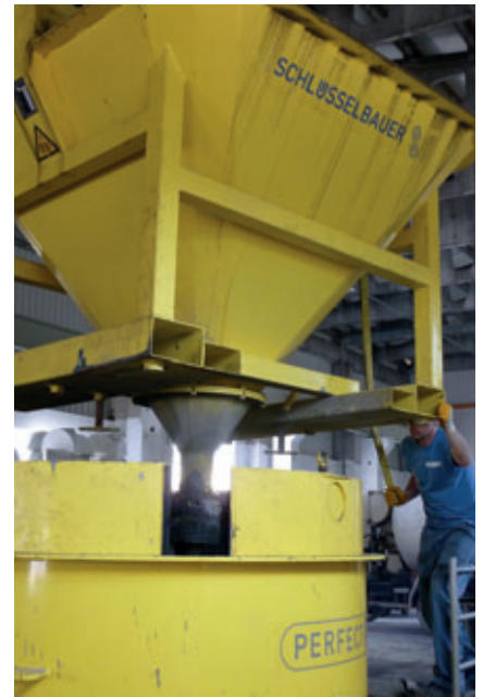
Werra-Baustoffwerk uses ready-mixed concrete to produce the manhole bases, which is poured using a crane track and a hopper
