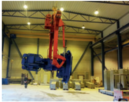
Turning with the turning spreader beam
