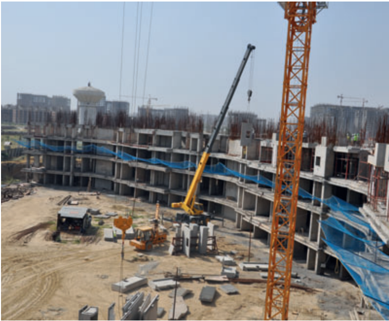
Construction site with precast walls and hollow-core slab
