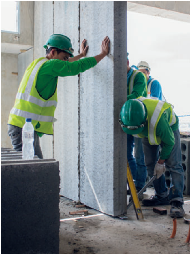
Acotec-wall installation
