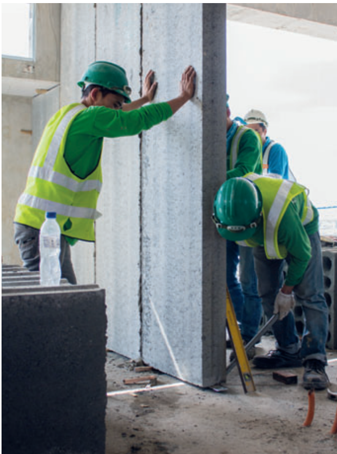
Acotec-wall installation
