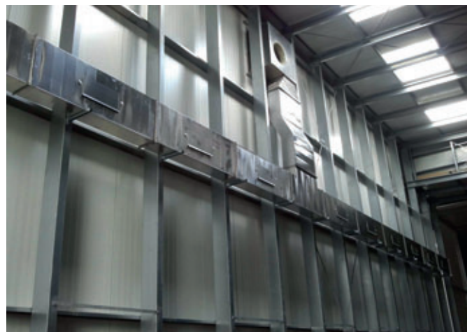
The stainless steel construction with an insulated housing guarantees a long service life, operational reliability and a constant high performance.
