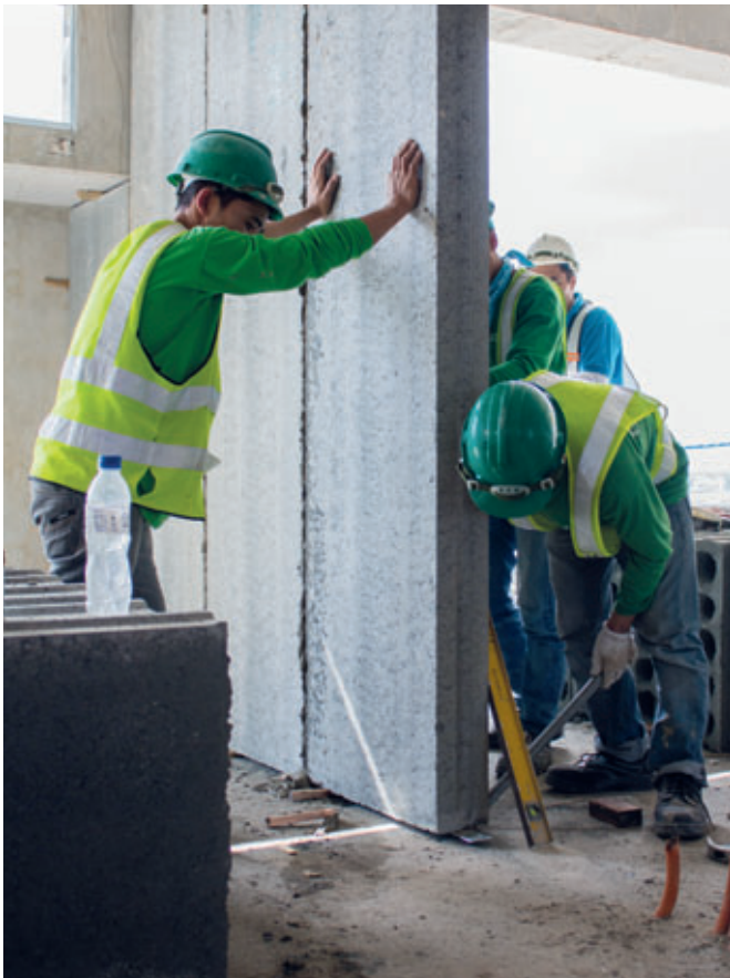
Acotec-wall installation
