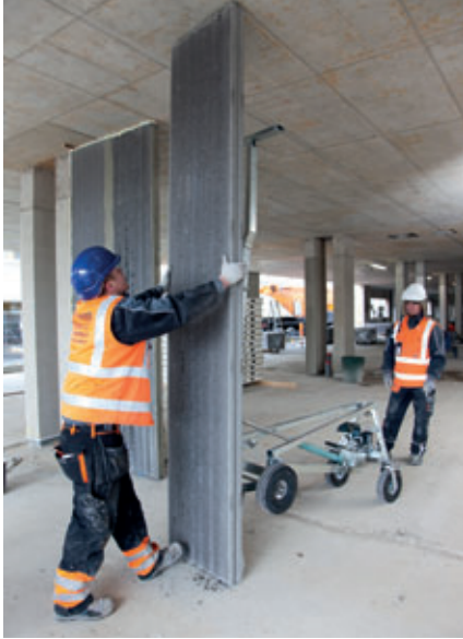
Acotec wall installation: A two men team installs 40-60 m 2 of Acotec wall in a workday.
