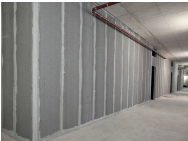
Long straight Acotec wall ready for finishing.
