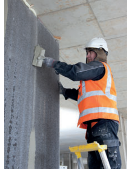
Finishing the joints.
