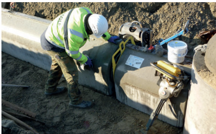
A link element is connected to the monobase with the same connectors as the pipe-pipe connection
