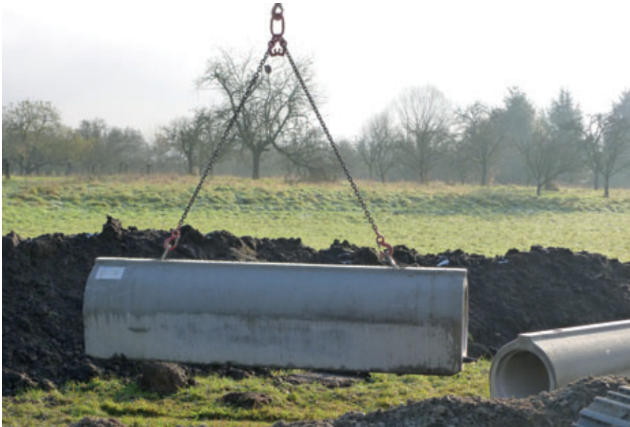
Simple and safe handling of the Perfect Pipes on the construction site with cast in lifting anchors
