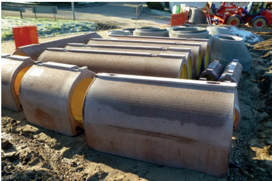
Perfect Pipe pipes with HDPE liner before installation in 3 m effective length, as an adaptor pipe with an individual construction length and as a 1 m link element
