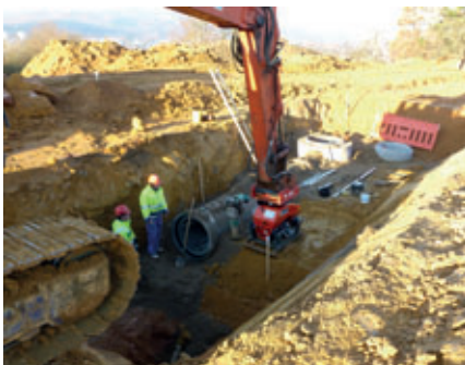
Rapid installation progress by simple and practical compression of the pipe zone
