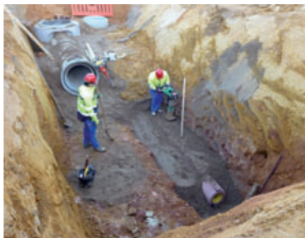
Rapid installation progress by simple and practical compression of the pipe zone
