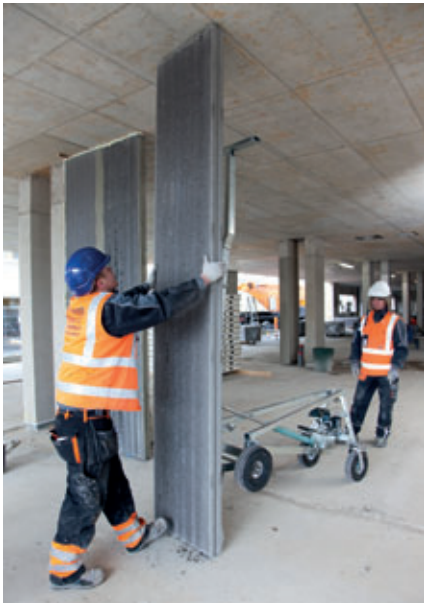
Acotec wall installation: A two men team installs 40-60 m 2 of Acotec wall in a workday.
