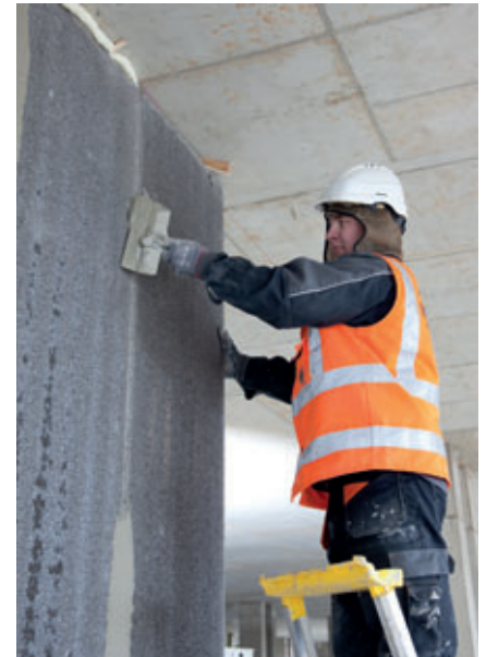
Finishing the joints.
