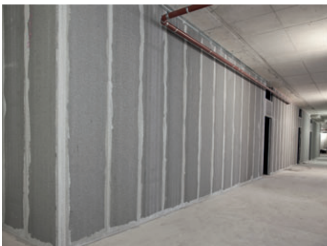
Long straight Acotec wall ready for finishing.
