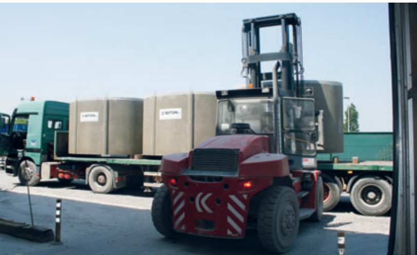
The finished concrete containers are loaded onto trucks for transport to the building site.
