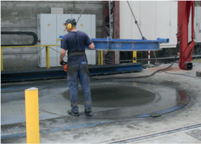
The pallet is automatically clamped to the filled and compacted mould.
