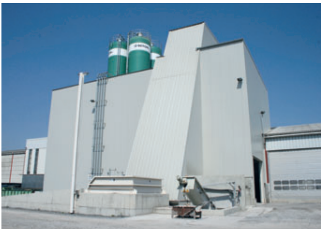
Ubo engineering b.v. built the new central mixing plant completely enclosed and located directly adjacent to the production halls.
