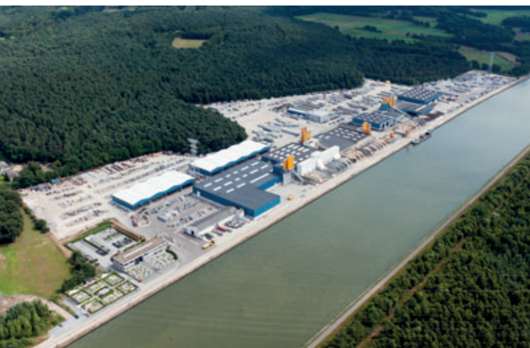
The 17-hectare Ebema works site in Zutendaal
