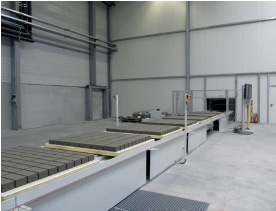
Transport system on the wet side
