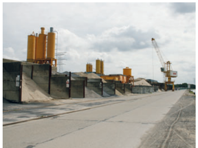
90% of the aggregates are delivered to Ebema by ship
