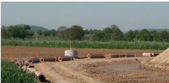
Pipe and manhole material are ready for installation.
