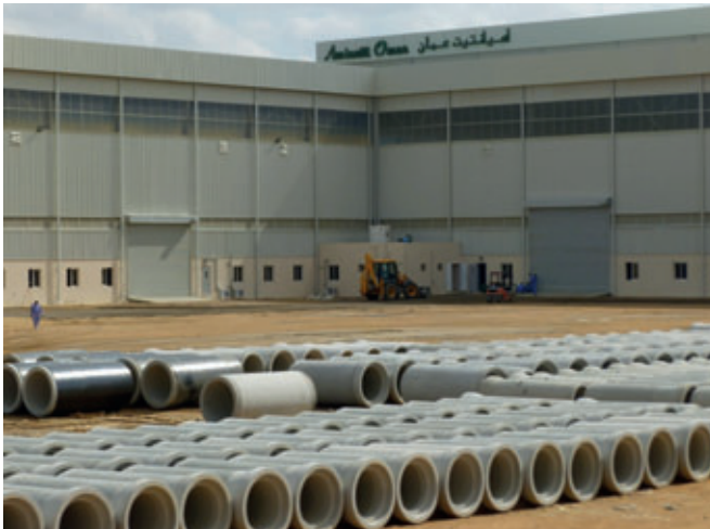
The most state-of-the-art concrete pipe facility in the Sultanate of Oman was opened by Amiantit Oman Concrete Products LLC in Autumn 2012.
