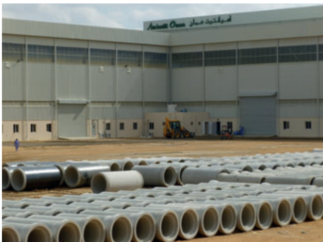
The most state-of-the-art concrete pipe facility in the Sultanate of Oman was opened by Amiantit Oman Concrete Products LLC in Autumn 2012.
