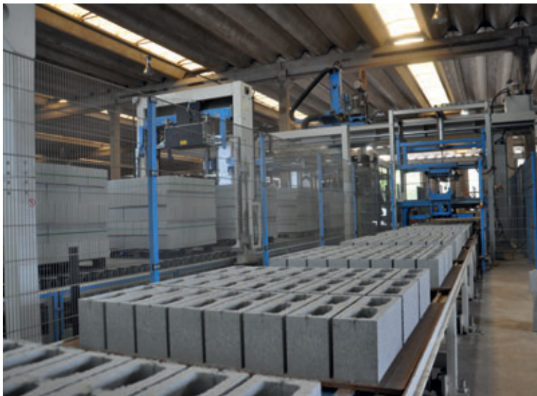
Walking beam conveyor on the dry side
