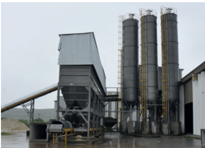
Dosing and mixing plant
