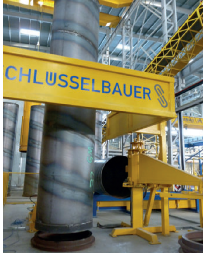
The sheet steel cylinder is automatically placed on a joint and concreted after the equipping of the mould for the manufacture of the internal lining of earth-moist concrete.
