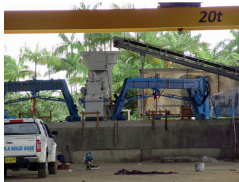
Installation of the plant
