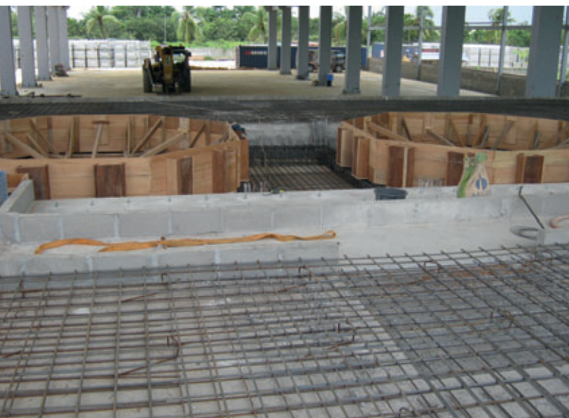
Preparing of foundation
