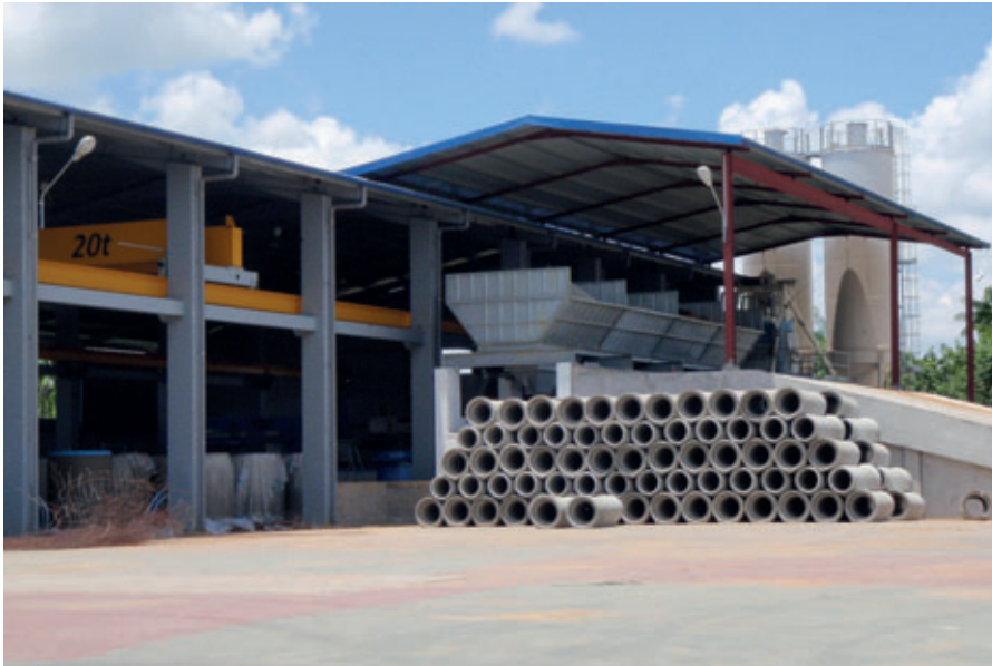
New concrete pipe making plant
