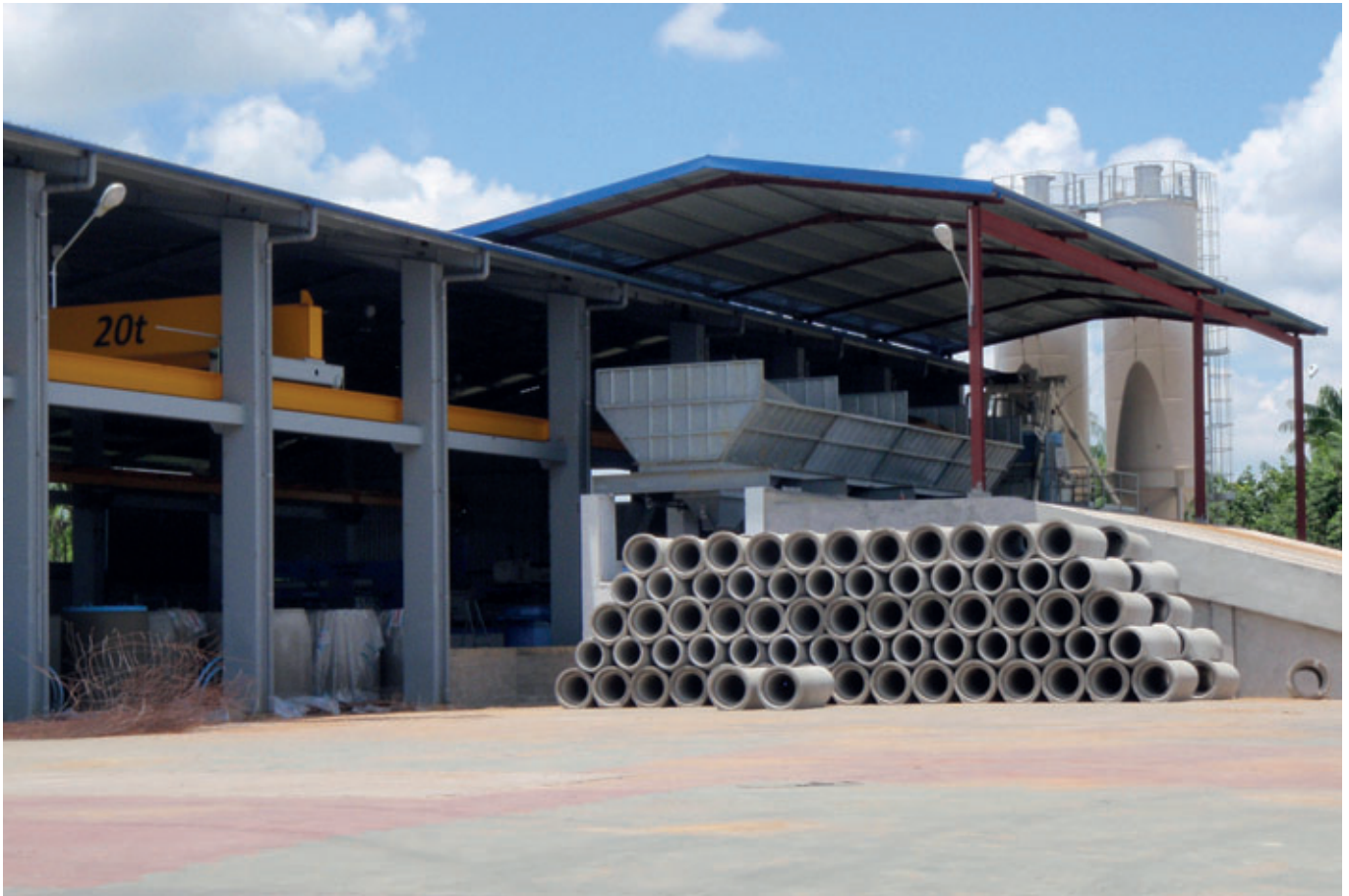
New concrete pipe making plant
