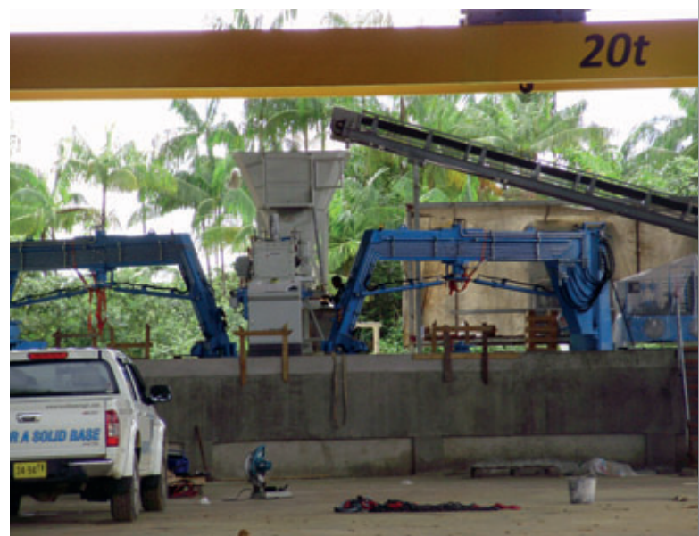
Installation of the plant
