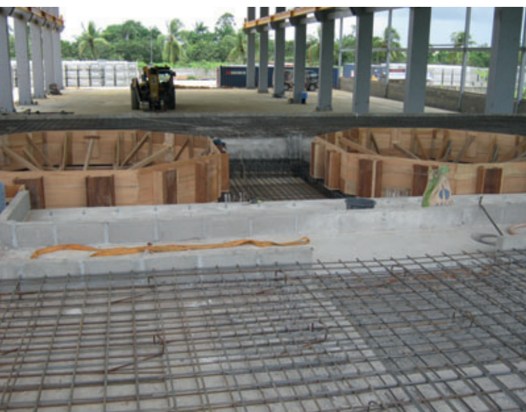
Preparing of foundation
