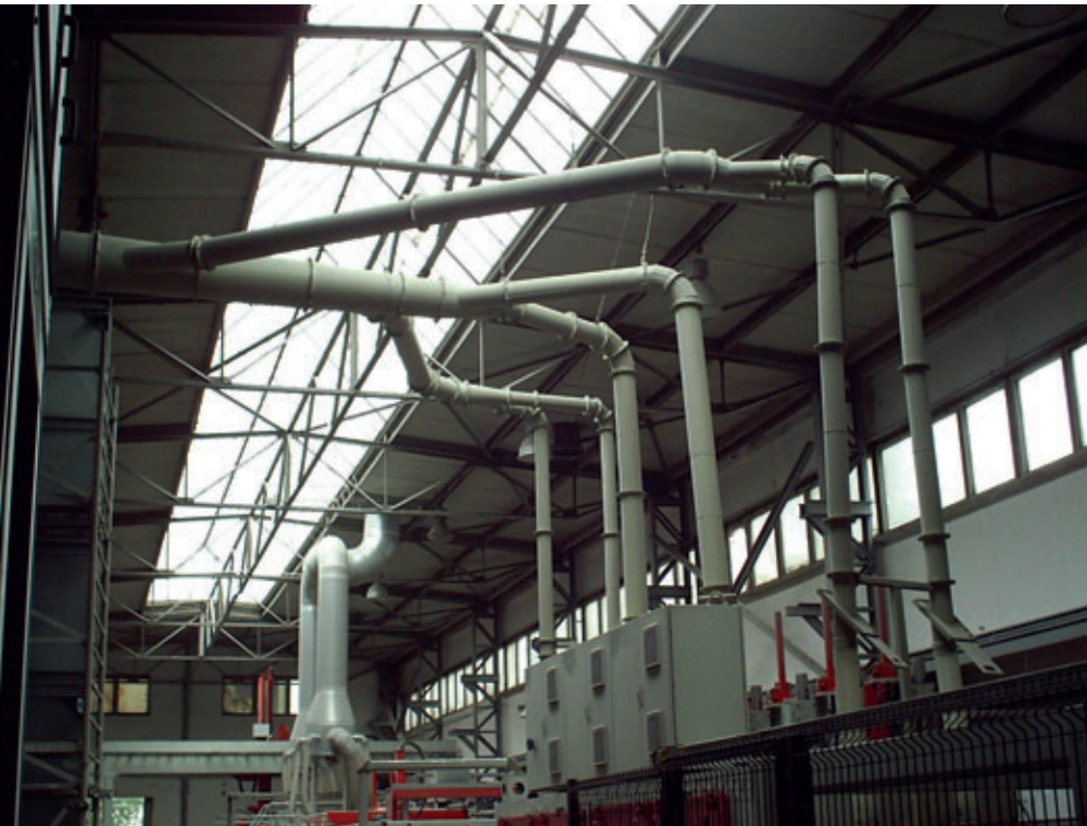
Piping to separately located suction plants
