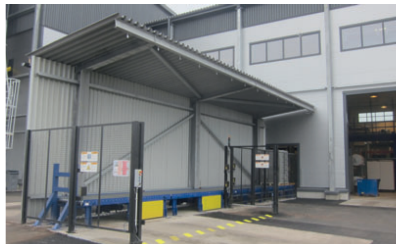
No corners were cut in Oitti where safety technology was concerned. All stations were planned and implemented to very high safety standards.
