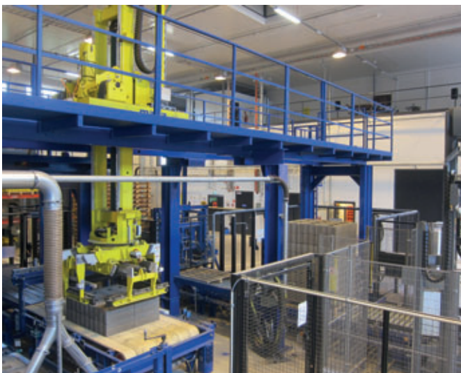
The second gripper robot takes up two block layers, which had been prepared by the layer doubler beforehand, and makes block packets out of them on the track located behind.
