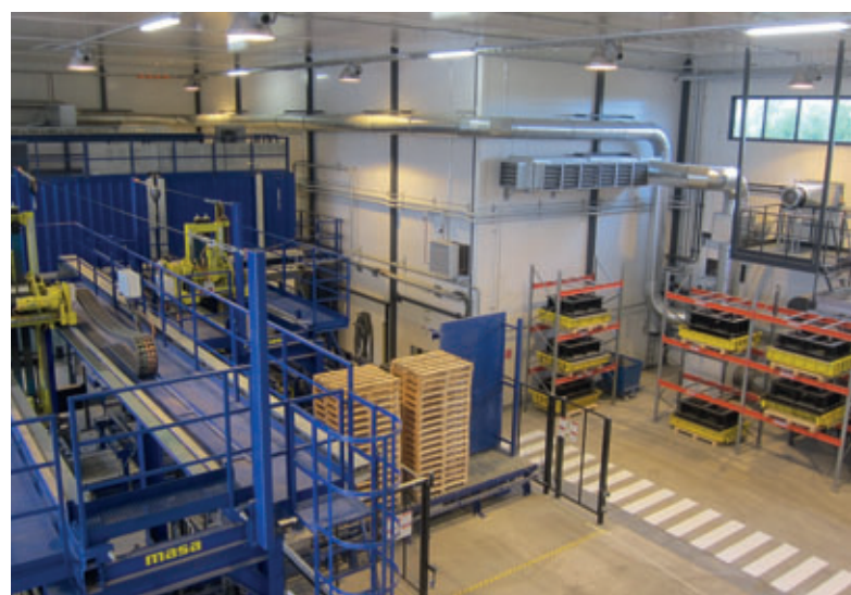
The winters in Finland are long and hard. In order to be able to produce continuously despite that, the complete hall has been lined with flame retardant insulating elements.
