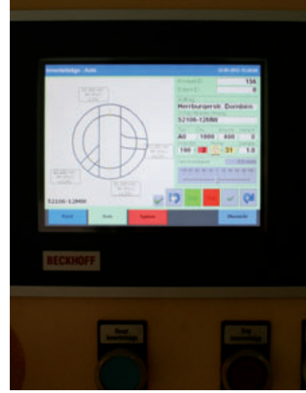
Operator guidance is provided via comprehensible displays on the individual workstations.
