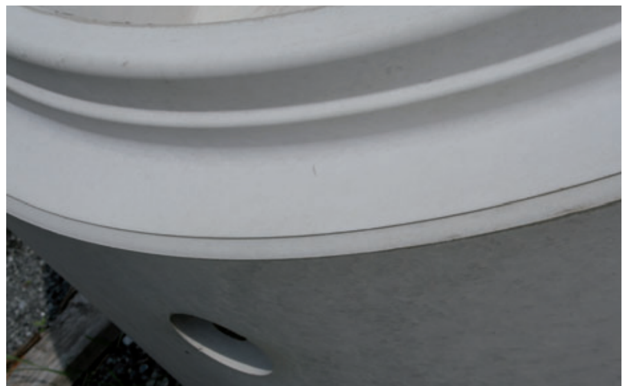
Visible product quality – the pre-assembled components manufactured with ready-mixed concrete from the Rhomberg concrete plant are convincing due to their flawless surface.
