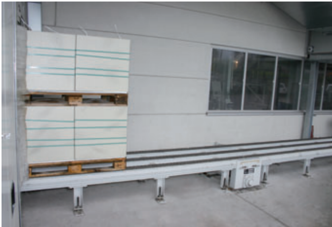
Figure 10: Packet transport to removal by fork lift truck
