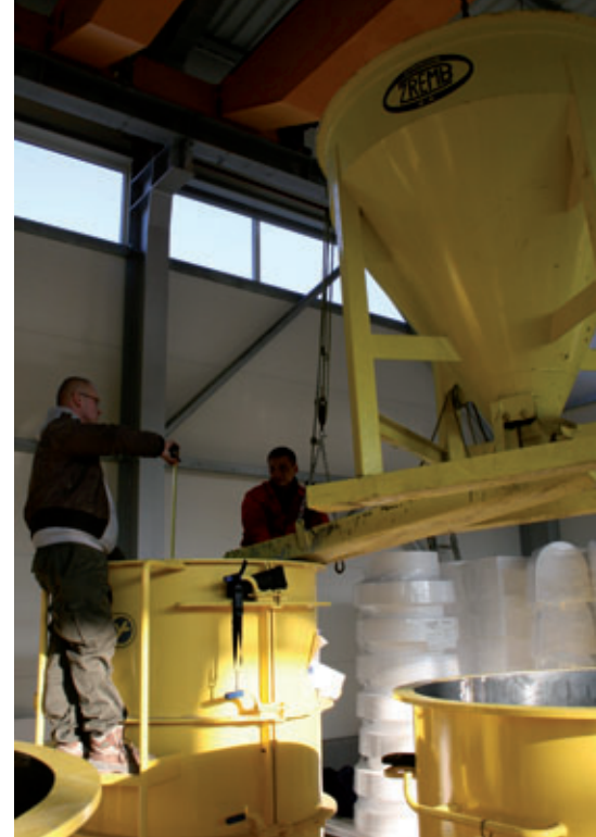
Pouring with bucket and crane track
