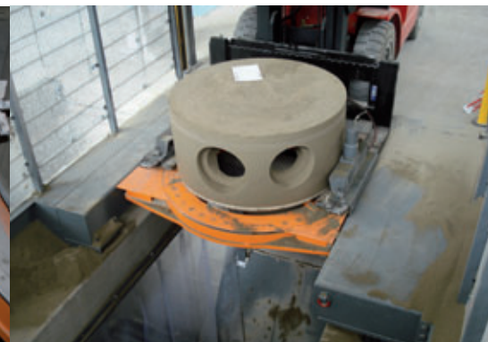
Removal of milled manhole base from the Primuss machine
