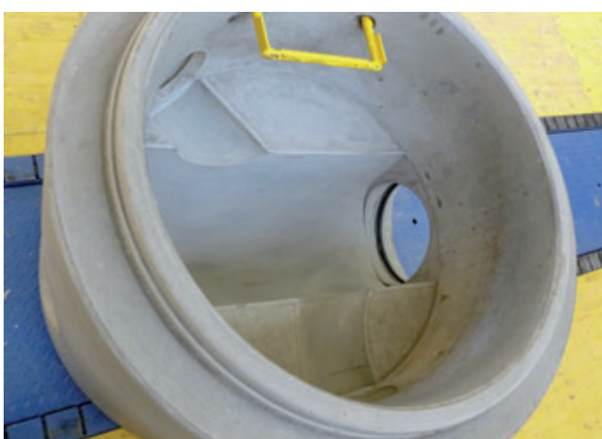
Finished manhole base with mounted step
