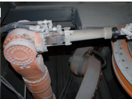
The milled material falls directly into the working pit, from where it is continuously removed by a conveyor.
