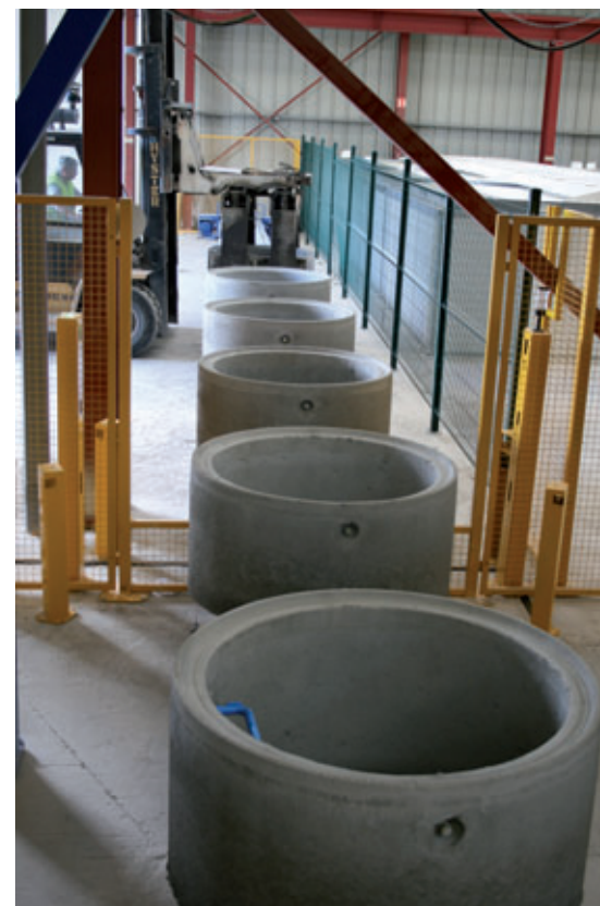
Transfer to the product conveyor belt. The concrete components leave the production hall in the next shift
