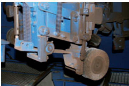
Steel brushes removing concrete residue from the pallets
