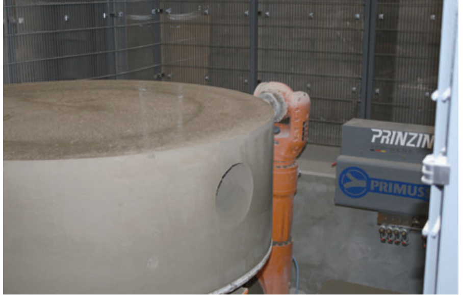
Milling the connections
