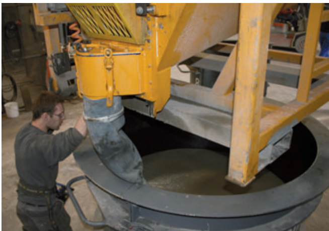
Carefully filling the casting mould with SCC
