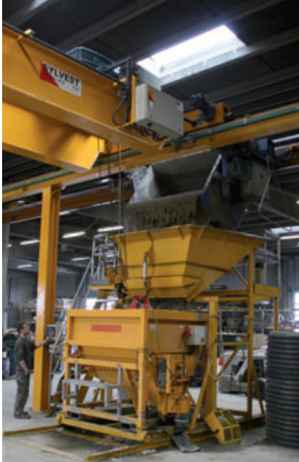
Transfer of SCC from the bucket conveyor to the concrete spreader
