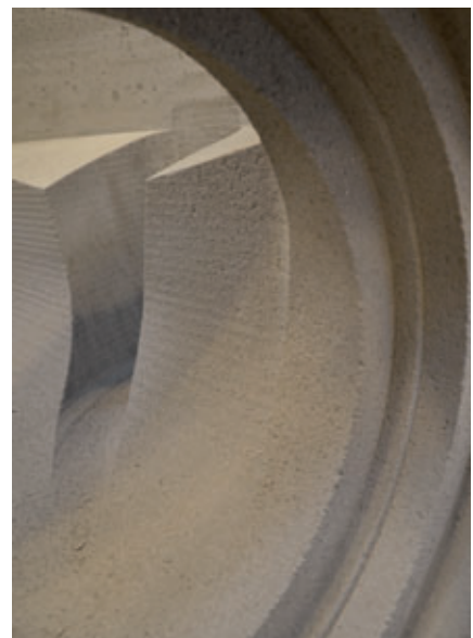
View of a milled manhole base section
