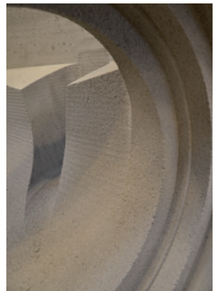
View of a milled manhole base section
