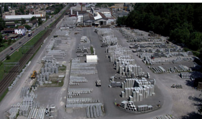
Creabeton Produktions AG company premises in Brugg, Switzerland
